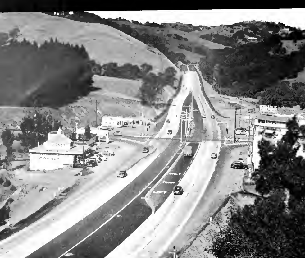
Orinda Junction on Sign Route 24, Oakland-Walnut Creek arterial, has full traffic signal control and channelization
